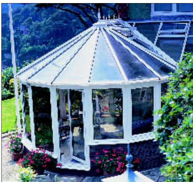
1.5 The roof system (see Figure 5) consists of a ridge beam and glazing bar sections extruded from aluminium to BS 1474 : 1987, material designation 6063-T6, glazed with 16 mm (three wall), 25 mm (five wall) or 35 mm (four wall) polycarbonate panels with co-extruded UV protection layer or 24 mm double-glazed sealed units that carry the BSI Kitemark BS 5713 : 1979.
