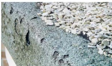
UV radiation and building movement can cause cracks, splits and blisters in traditional felt. Failure can also result from poor design or installation.
