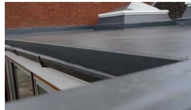
Aesthetically pleasing membrane coated edge trims are available in a choice of colours. These provide strong weather resistant roof edges.
