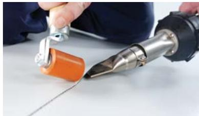
Sarnafil roofing membrane are permanently fused together by hot air welding at joints and on details. This ensures a durable and watertight finish.
